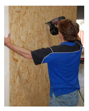
9. Repeat the process for the next and subsequent SIP panels ensuring that either mastic or expanding foam is applied to both the horizontal sole plate and the vertical joining spline timbers. Nail the joining spline at the same centres as the sole plate on both inside and outside of the building.
