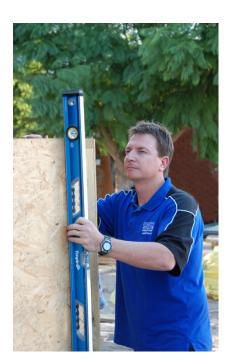
8. Nail the SIP panel through the OSB skins into the sole plate at no more that 150mm centre with 51mm ring shank nails on both inside and outside of the building. Check with engineer's detail for nail schedule. These nails are also used to nail the SIP panels together on the joining splines on both inside and outside of the building as per engineers spec.
