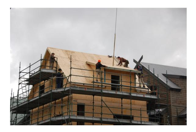
21. The SIPS structure must be papered with a breathable membrane and this must be installed as per the manufacturers guidelines. The breathable paper must be fixed to the kit as per the manufacturers guidelines.
