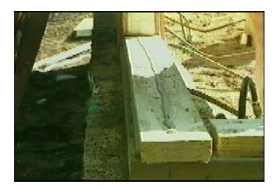
6. Lift the first panel into position, working from one corner of the slab. Panels are usually lifted into place by mechanical means, but can be man handled if only 1200mm x 3800mm x 162mm panels or smaller.
