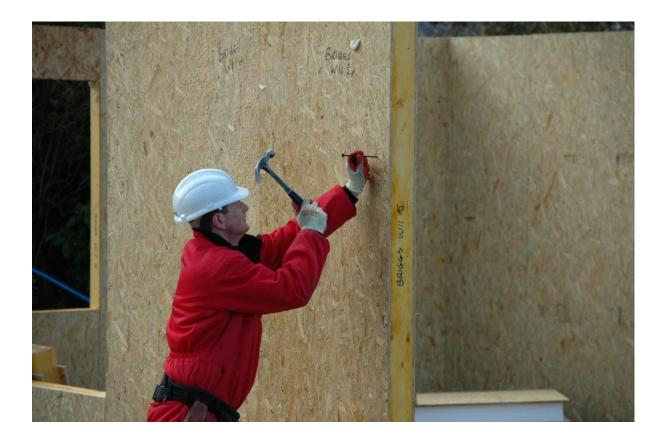
10. Continue to install the SIPS until all the wall SIPs are in position, continually checking the plumb and level of the panels as you progress.
